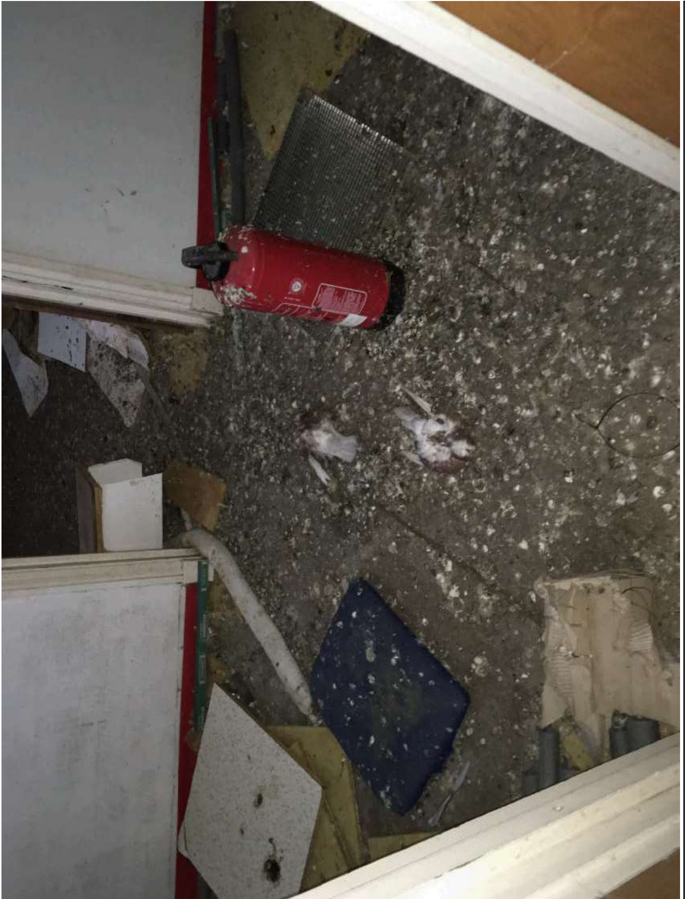
Image showing the internal condition of the building - image 3
