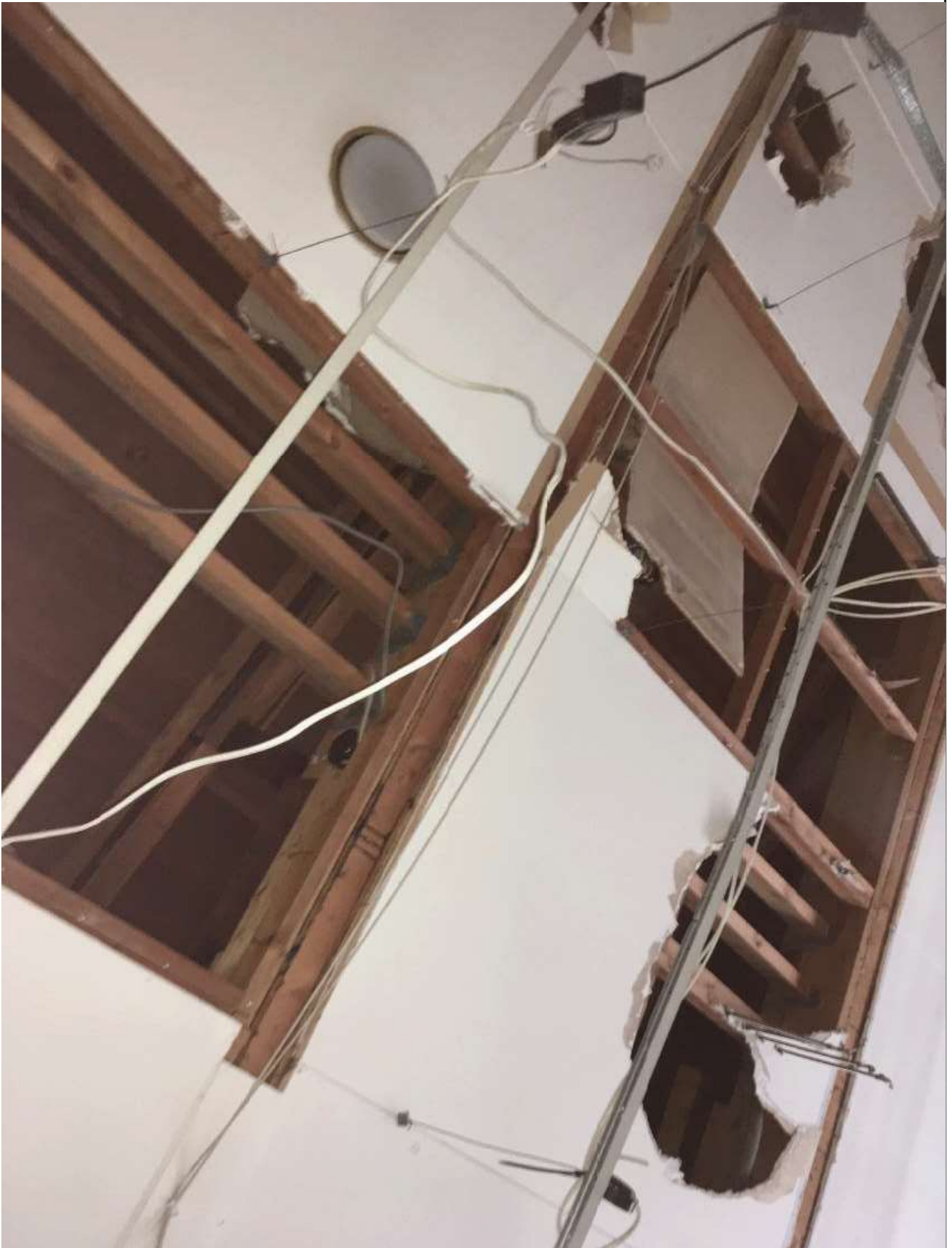
Image showing the internal condition of the building - image 7
